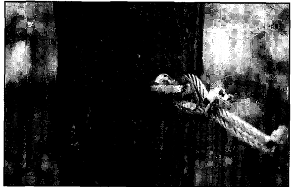
Figure 1. The crown anchor is mechanically well done, but is it really the best solution for the tree?
