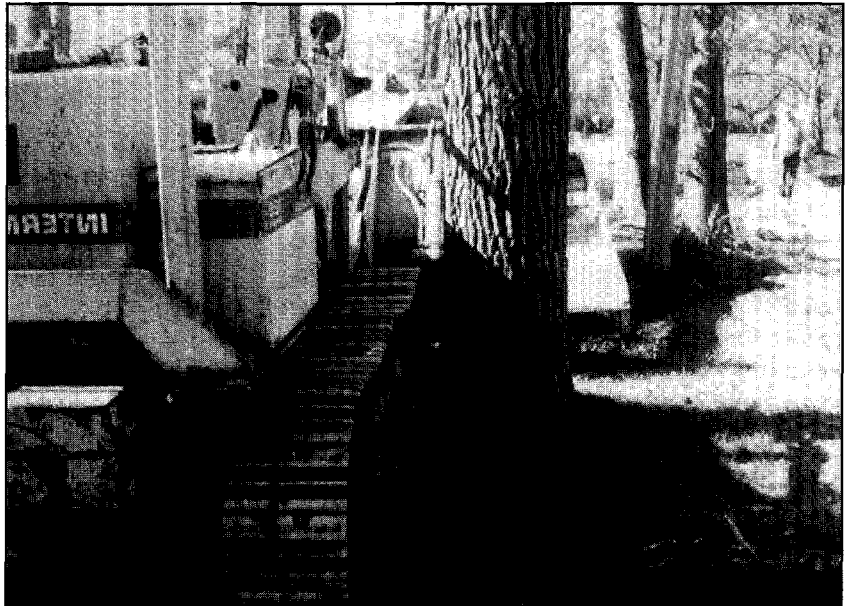
Figure 1. Heavy equipment parked on parkway compacts parkway tree root zone area and can injure the tree trunk.
