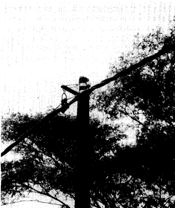
Figure 6. Aerial cable system.
