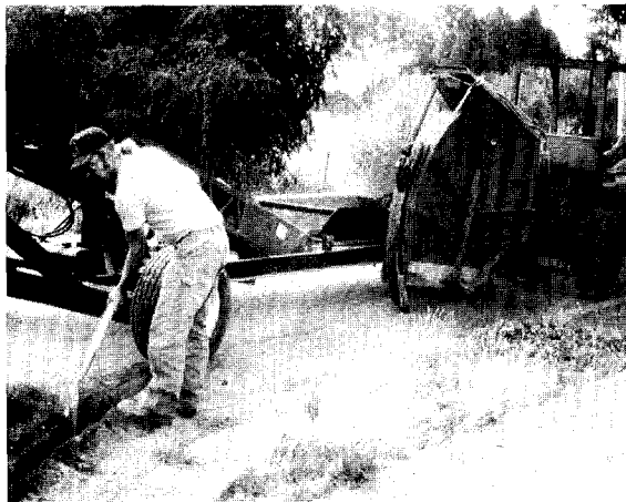
Figure 8. Wheel trench construction.
