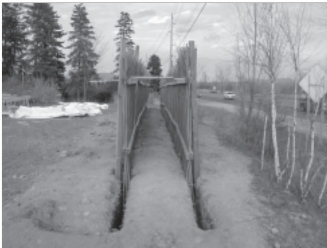
Figure 2. Stems are assembled tightly in a wooden frame and installed upright in two trenches set 1.2 m (4 ft) apart.
