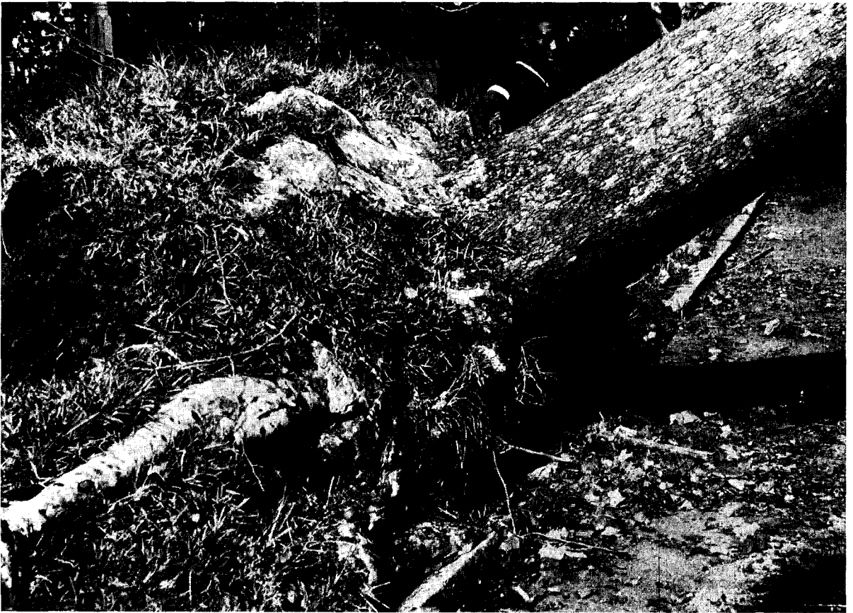
Figure 1. The roots of this 30" diameter sycamore ran parallel to the street and could not support the tree against winds coming from other directions.
