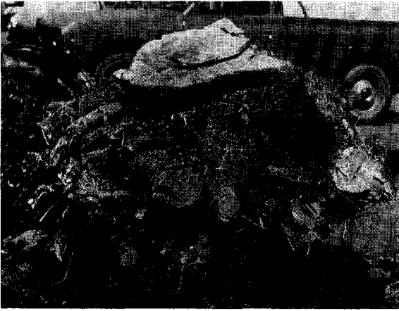
Figure 1. Norway maple stump and root system with several girdling roots visible.
