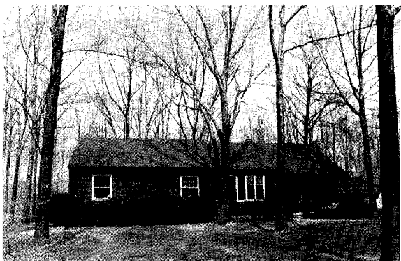
Figure 2. The house shown in Figure 1 as it appeared at midday in March. Note that bare trees still shade substantial portions of the house.
