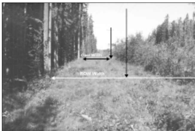
Figure 2. Clear width: The distance measured on the ground from the trunks at the tree line to the nearest conductor.
