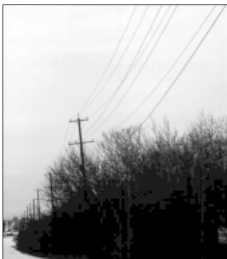
Figure 1. New growth has been “burnt off” from occasional line contact (center of photo).
