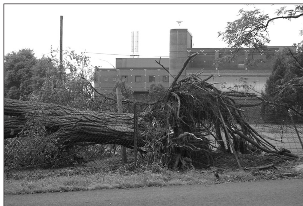
Figure 6. Tree failure resulting from saturated soil conditions during tropical storm Ernesto, in 2006.
