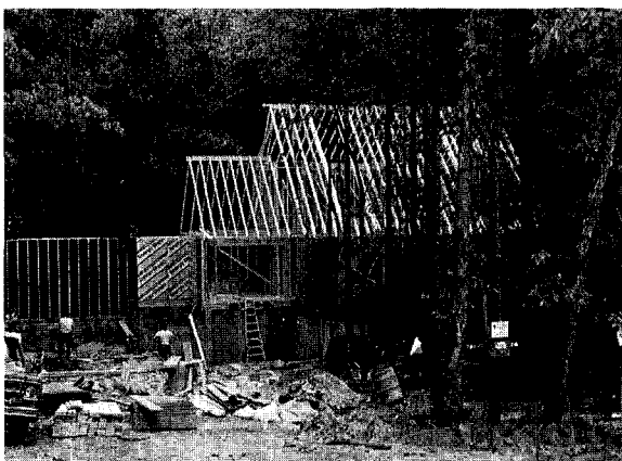
Figure 1. Protecting the roots of trees during construction is as important as protecting the trunk. The shade over this new home may be shortlived because of the extensive soil disruption around the trees.
