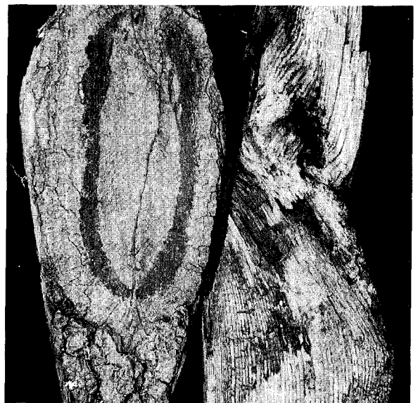
Figure 8. Improper flush cut on the same tree as shown in Figure 7. The cut was made 30 years ago. Note the advanced decay above and below the cut. The wound appeared closed, but there was space between the long crack. The space provided enough of an opening to make conditions perfect for the decay-causing fungi.
