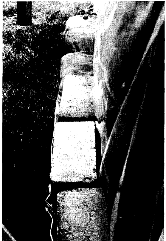
Figure 2. Two possible methods of sealing woodpiles are shown here; placing sandbags or concrete blocks on the excess polyethylene.
