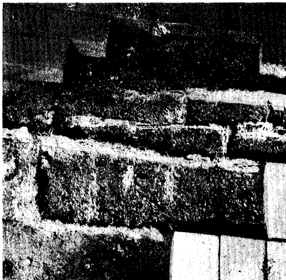
Figure 11. Roots growing in crevices of bricks. There was no oxygen below the bricks which overlie a compact clay on the N.C. State University Campus. Tree roots commonly follow cracks and crevices or air passages under pavement.
