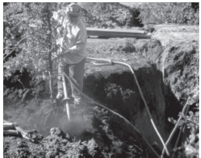
Figure 1. After 4 years, root systems of coast live oak were fully excavated using a pneumatic excavation tool (Air-Spade®), backhoe, and jackhammer.
