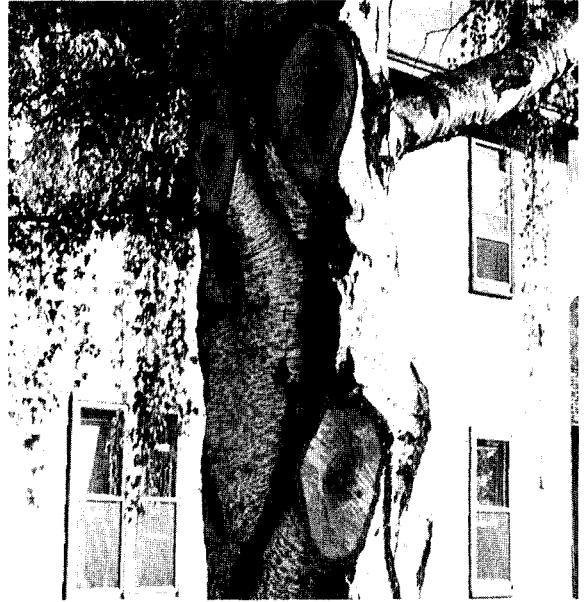
Figure 12. Power equipment can make large cuts with ease but these callus slowly allowing secondary organisms to enter.
