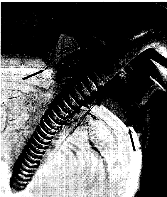
Figure 9. The hooked end of this lag injured the bark and caused a large dead spot (arrows). Decay developed around the screw. The dead spot slowed the compartmentalization process. The lag was inserted 8 years ago.
