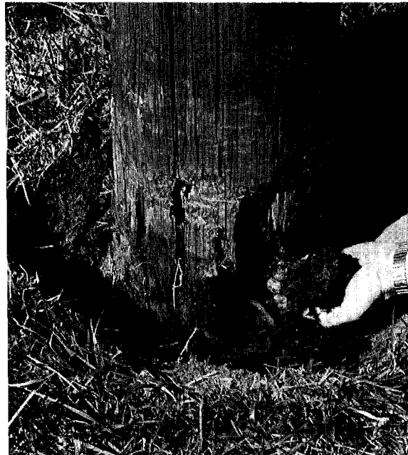
Fig. 1. External and internal decay just below groundline on a southern yellow pine pole.
