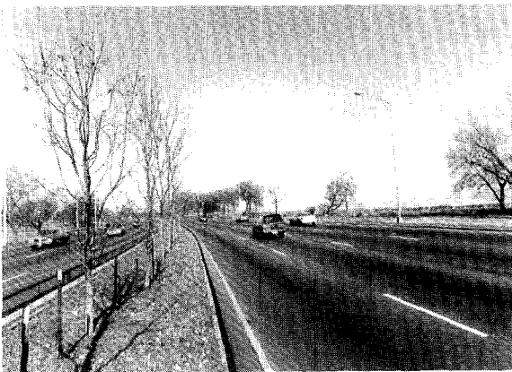
Figure 1. Narrow median planter along Lake Shore Drive, Chicago, with Lake Michigan in the right background. The planter is raised 0.8 m (2.5 ft) above the roadway. Photo credit: Jim Nachel
