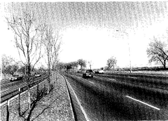
**Figure 1. Narrow median planter along Lake Shore Drive, Chicago, with Lake Michigan in the right background. The planter is raised 0.8 m (2.5 ft) above the roadway. Photo credit: Jim Nachel**
