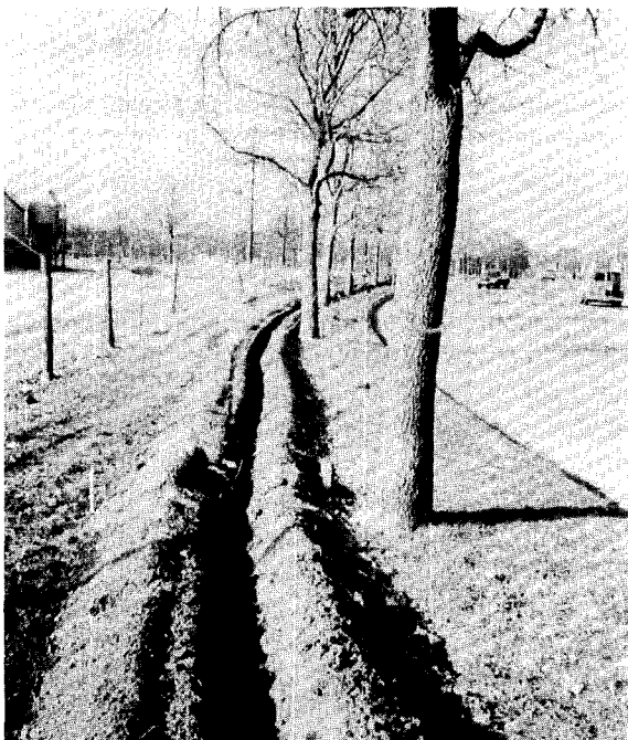
Figure 1. Trenching alongside hackberry trees on the University of Illinois campus in 1987.
