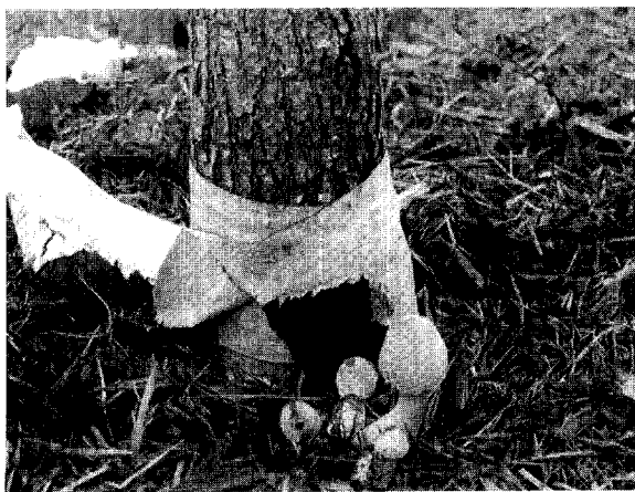
Figure 5. A potentially lethal combination at the base of this tree; tree wrap held in place by a deep mulch layer. The bark and paper wrap were water-soaked and stained, and mushrooms growing on the mulch were evidence of the saturated condition.
