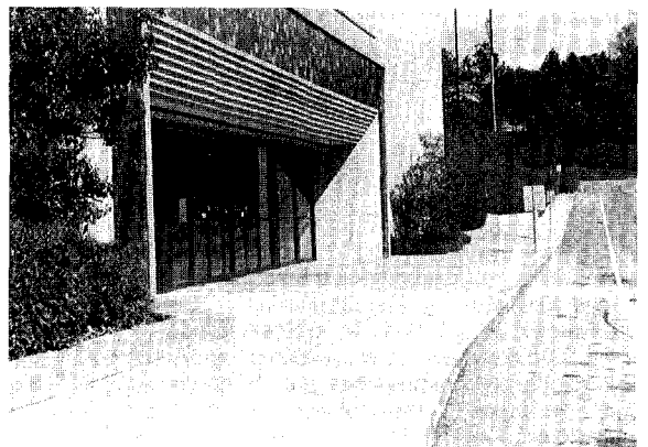
Figure 2. Highly visible entrances to buildings are reassuring to parking lot users. Vegetation can help define and locate the doors, but it should not interfere with the view from the lot to doorway or from the doorway into the lot.
