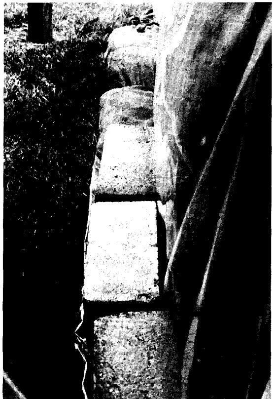
Figure 2. Two possible methods of sealing woodpiles are shown here; placing sandbags or concrete blocks on the excess polyethylene.
