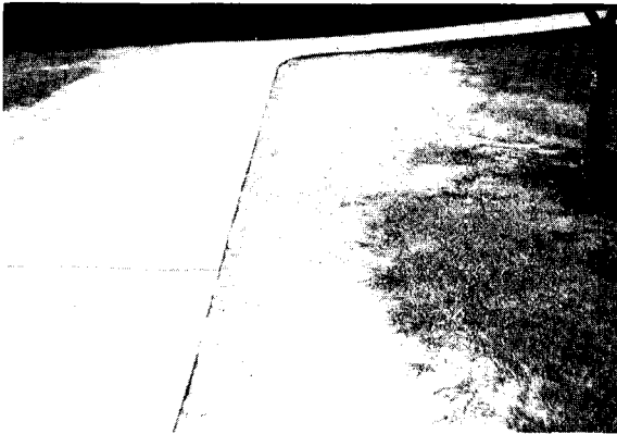
Figure 1. Turf damage from deicing salts used on the sidewalk.
